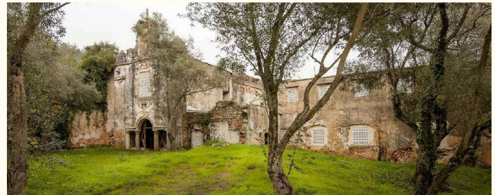
After the intervention
