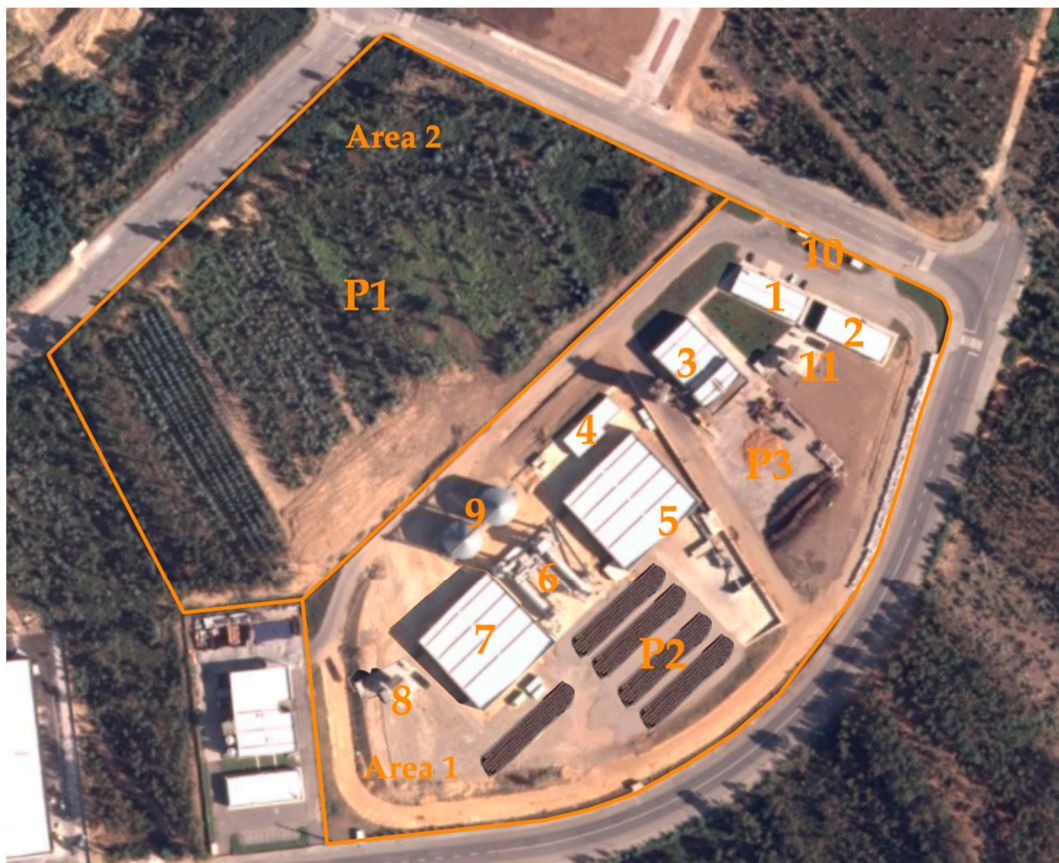
Figure 1. Advanced Fuel Solutions SA (AFS) facilities, where Area 1 corresponds to a plot of land of 42,000 m 2 and Area 2 corresponds to a plot of land of 40,000 m 2 . P1 corresponds to a 2500-m 2 raw material storage park that supports the experimental pilot unit; P2 corresponds to a raw material storage park of approximately 7500 m 2 that serves for the production support stock; and P3 corresponds to a 40,000 m 2 storage park that serves as a strategic storage stock, with a capacity for 3 months of production. (1) Social building; (2) R&D department; (3) pilot-industrial scale production unit; (4) maintenance building and parts warehouse; (5) raw material pre-processing section; (6) biomass drying and torrefaction unit; (7) densification section; (8) armed fire network of the industrial scale production unit; (9) finished product silos; (10) ordinance and scale; and (11) armed fire network of the pilot-industrial scale production unit.
