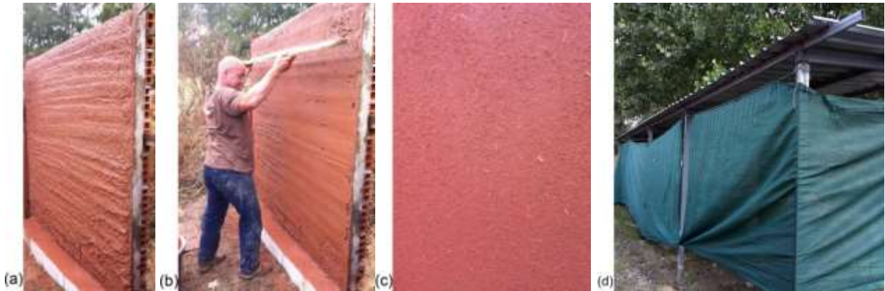
Fig. 2 Application of the earth plaster: (a) after mechanically application, (b) manual levelling and (c) finished surface; (d) protection of the experimental walls
